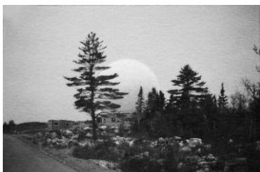
I took this picture of Mill Village I during the installation of Mill Village II in 1968. At the time of the MVI construction, during the early days of satellite communication many of the antennas used radomes (including the AT&T stations in Andover, Maine and its twin at Plumeur-Badou in France) whereas the British one at Goonhilly did not. In time, radomes fell out of favour. At Mill Village, therefore we had an example of each type. MVI (with radome) and MVII (without)
