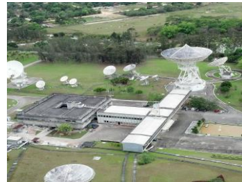
Here's a recent photograph Mike Morris found on-line of the earth station facility at Tangua. Obviously, it has changed a lot since 1968. I'm not sure which is the original antenna. I think it's the one in the foreground. The other big one (in the background) features beam waveguide which came along a lot later.
